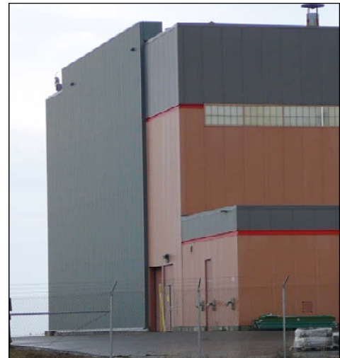
Military hangar with SolarWall system integrated into the façade.
