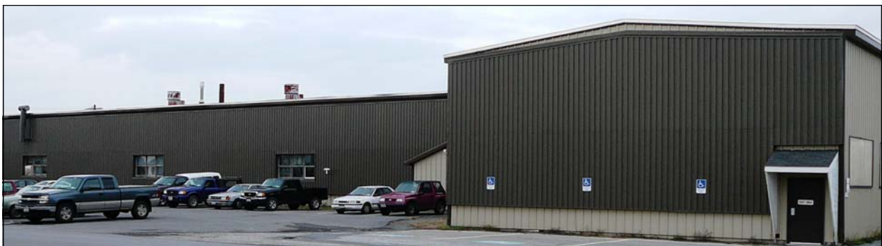
Dark bronze SolarWall system on a vehicle maintenance garage at Fort Drum.
