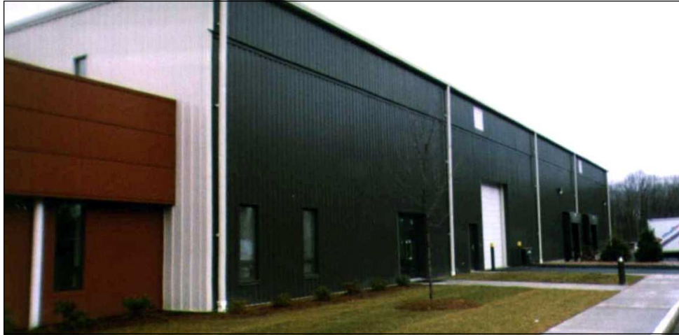
The completed SolarWall® system on Steeltech's warehouse
