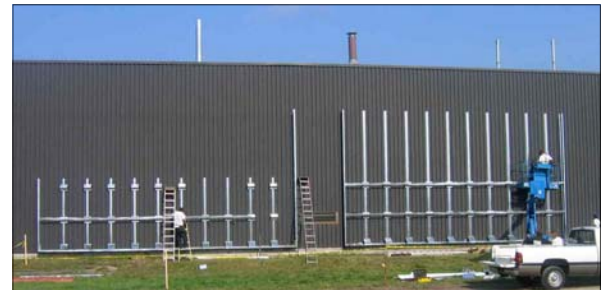
Above, the SolarWall® framing during construction
