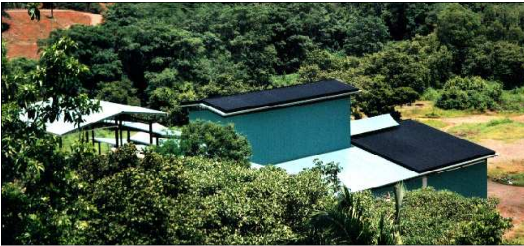
A black SolarWall® system over two roof sections at a new beneficio in the coffee-drying region of picturesque Sona, Panama.
