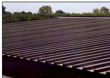
Roof mounted SolarWall system producing high quality "Solar Dried" walnuts
