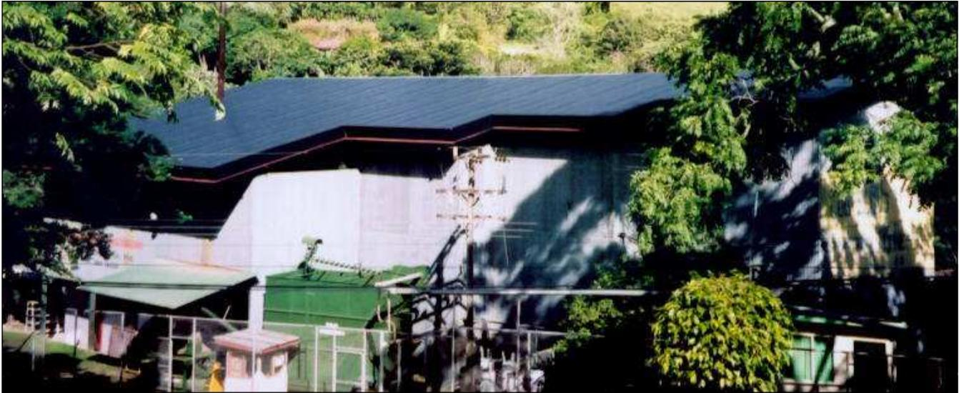
*A black roof mounted SolarWall® crop drying system used for coffee in Tilaran, Costa Rica*
