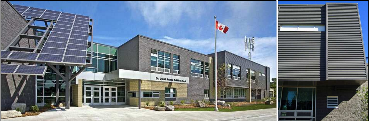
The front of the LEED® Platinum Dr. David Suzuki School and a close-up of the SolarWall® system
