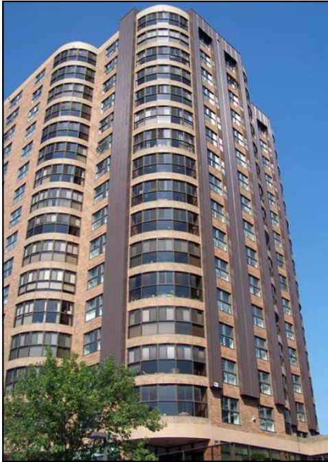
Left, Fred Douglas Place's SolarWall® solar air heating system designed to compliment the existing brick facade Above, Close-up view of three of the SolarWall columns
