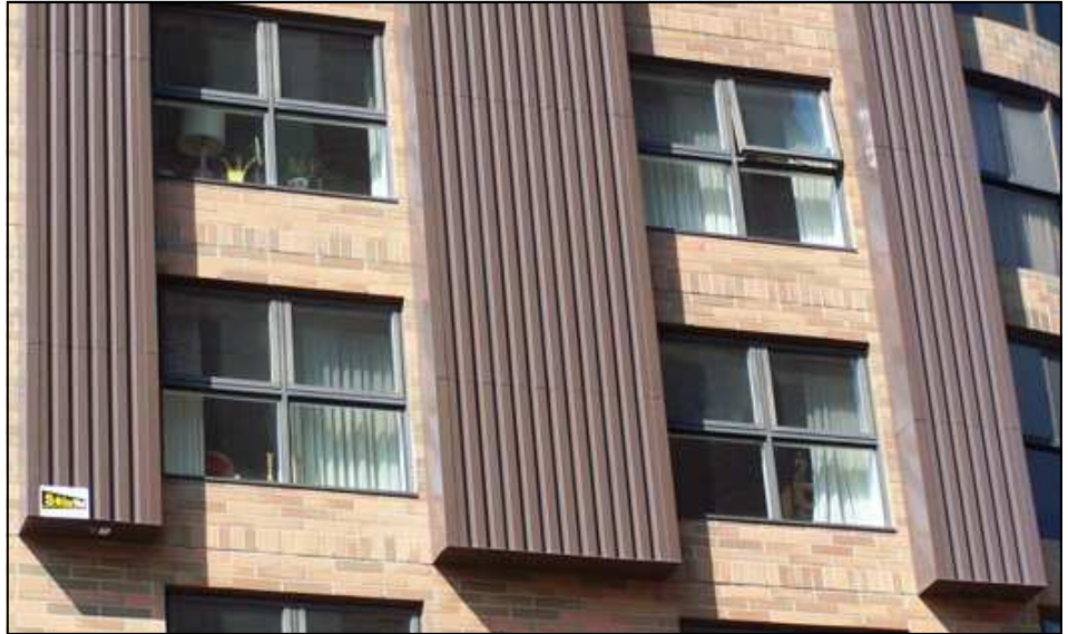
Left, Fred Douglas Place's SolarWall® solar air heating system designed to compliment the existing brick facade Above, Close-up view of three of the SolarWall columns
