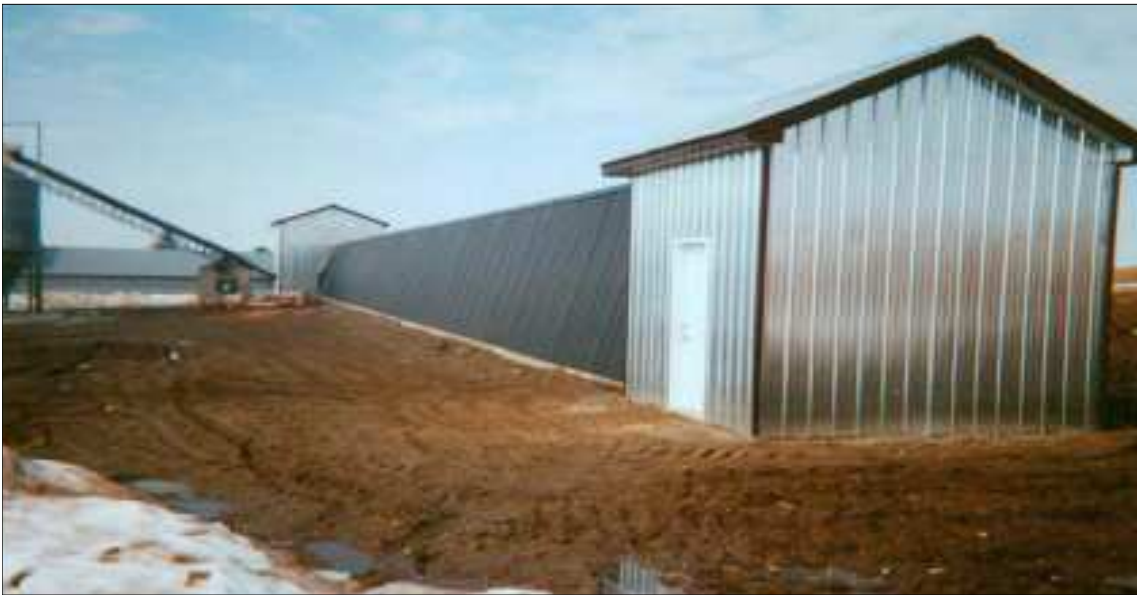
Left, SolarWall® installation at Gelé Chicken Farm, Cookshire Quebec, Canada
