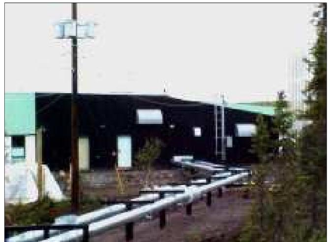
*SolarWall system installed in a permafrost climate*
