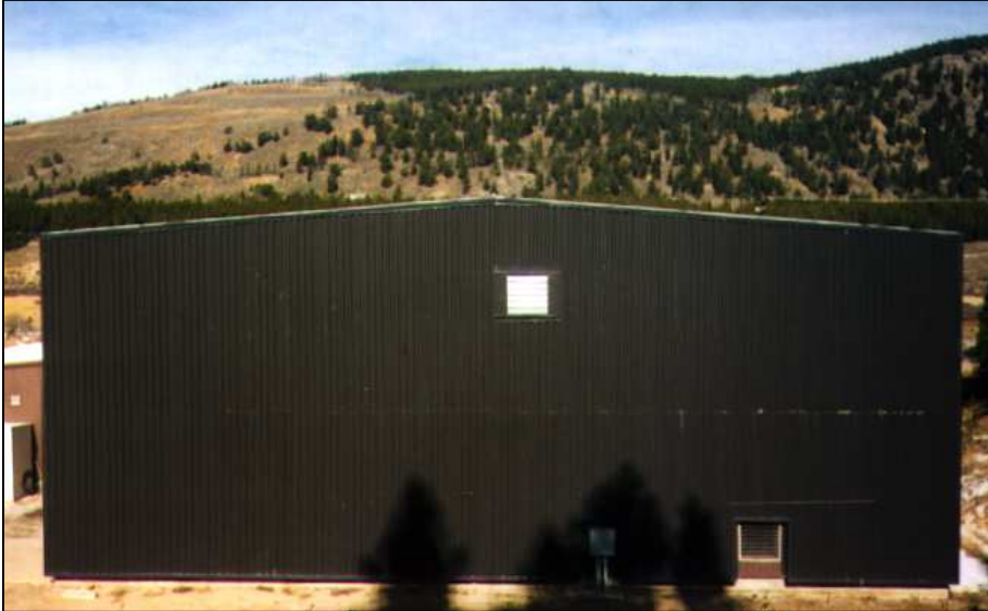
Left, a close up of the SolarWall solar air heating system installed at the Leadville Water Treatment Plant in Colorado. Top, angled view of the SolarWall and the rest of the water treatment facility.
