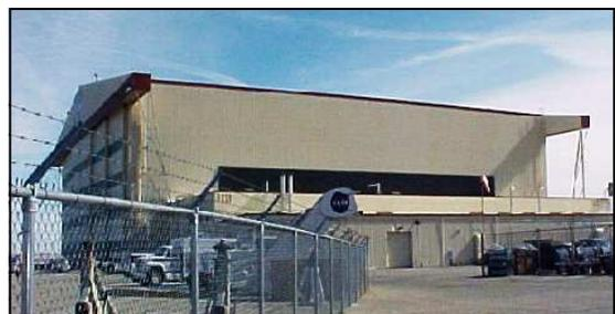
*Bronze SolarWall<sup>®</sup> system on the hangar heats incoming ventilation air*
