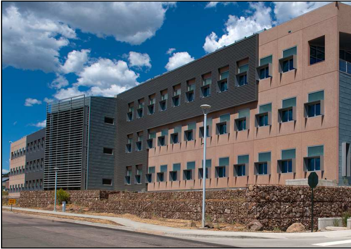
NREL's LEED® Platinum Plus Research Support Facility showcasing innovative green technologies such as the SolarWall® solar air heating system (above; the two south facing charcoal SolarWall® systems)
