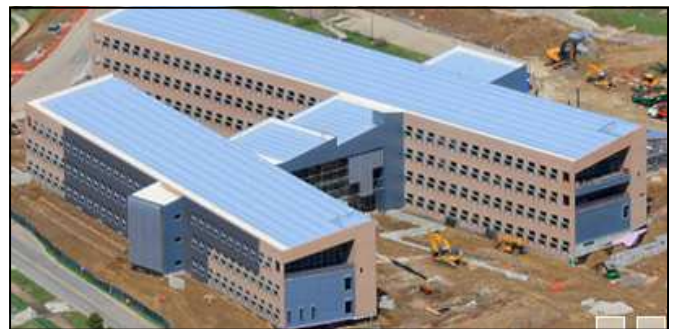
Aerial view of NREL's Research Support Facility, the two SolarWall systems are visible in the bottom left of the photo
