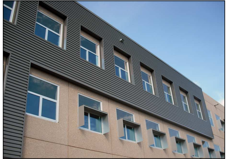
NREL's LEED® Platinum Plus Research Support Facility showcasing innovative green technologies such as the SolarWall® solar air heating system (above; the two south facing charcoal SolarWall® systems)
