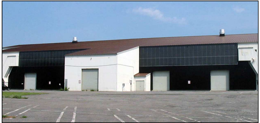
Above; photos of the SolarWall® 2-Stage solar air heating systems at Plattsburgh International Airport.
