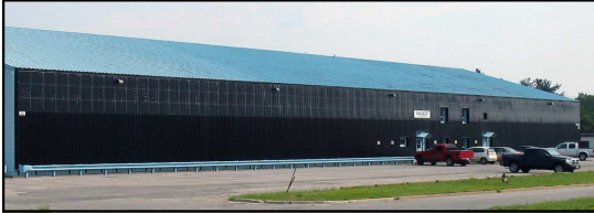
Above; photos of the SolarWall® 2-Stage solar air heating systems at Plattsburgh International Airport.
