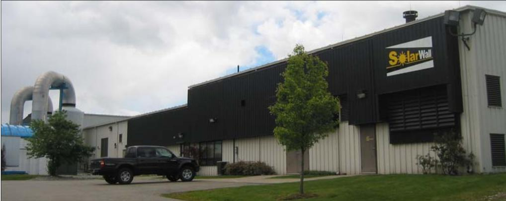
*Black SolarWall® panels installed on Wall 1 of the Rockland County Co-Composting Facility, located in the town of Ramapo, New York.*
