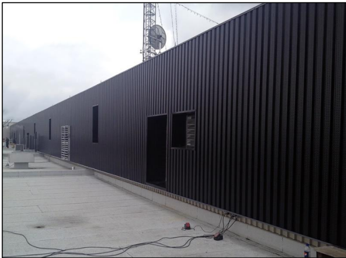
The Sherbrooke University Hospital SolarWall® solar air heating system located in Quebec, Canada.
