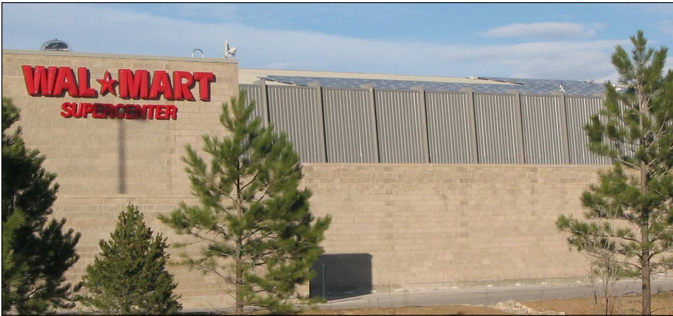
Grey SolarWall® panels on the south wall of Wal-Mart's new Denver-area Supercenter. The architectural "fins" were incorporated into the design to give the wall a unique appearance.
