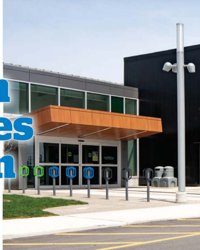
The new Waterloo Public Library features a black solar air heating system.
