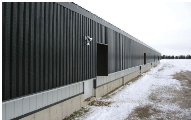
Before and after images of a SolarWall installation showcasing the transformation.
