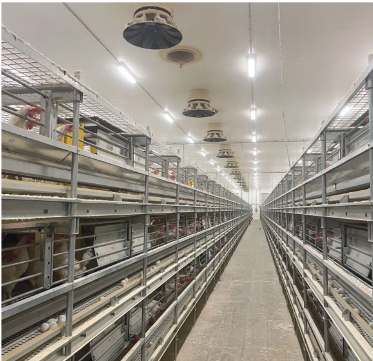
Ben Entz's SolarWall system channels fresh, pre-warmed air into powered inlets.
